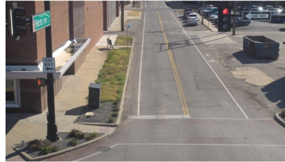
Webster Avenue Road Diet south of Main St
