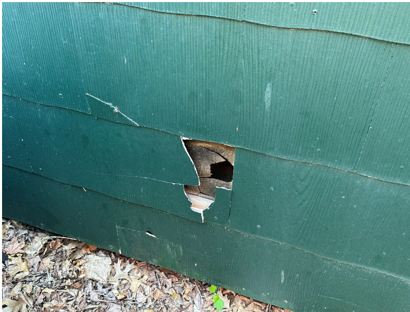
Damaged siding on north side of home
