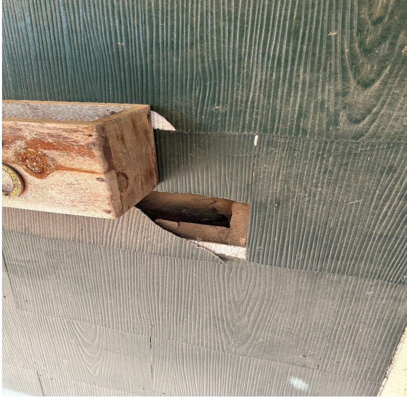
Damaged siding on porch
