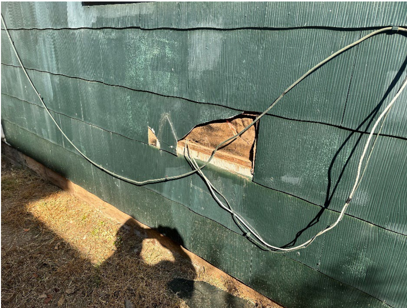
Damaged siding on south side of home
