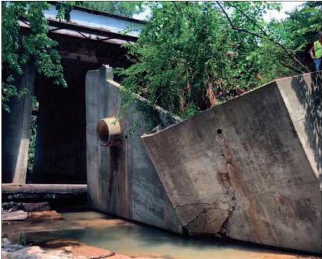
Figure 5: Failure of Wingwall on Imhoff Rd Bridge
