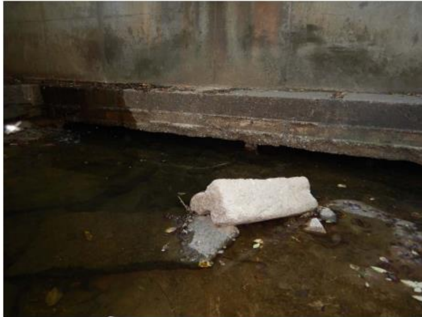
Figure 4-2: Undermining of the southeast wingwall of the structure at Imhoff Road
