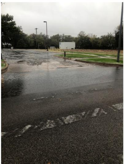
Water ponding in gutter line during rain events
