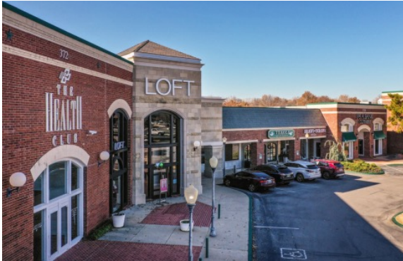
Brookhaven Village Building E
