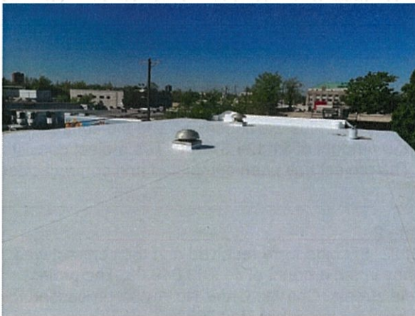
Roof membrane completion
