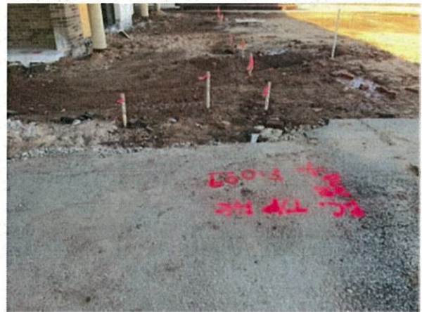
Marking For Underground Electric Sleeves
