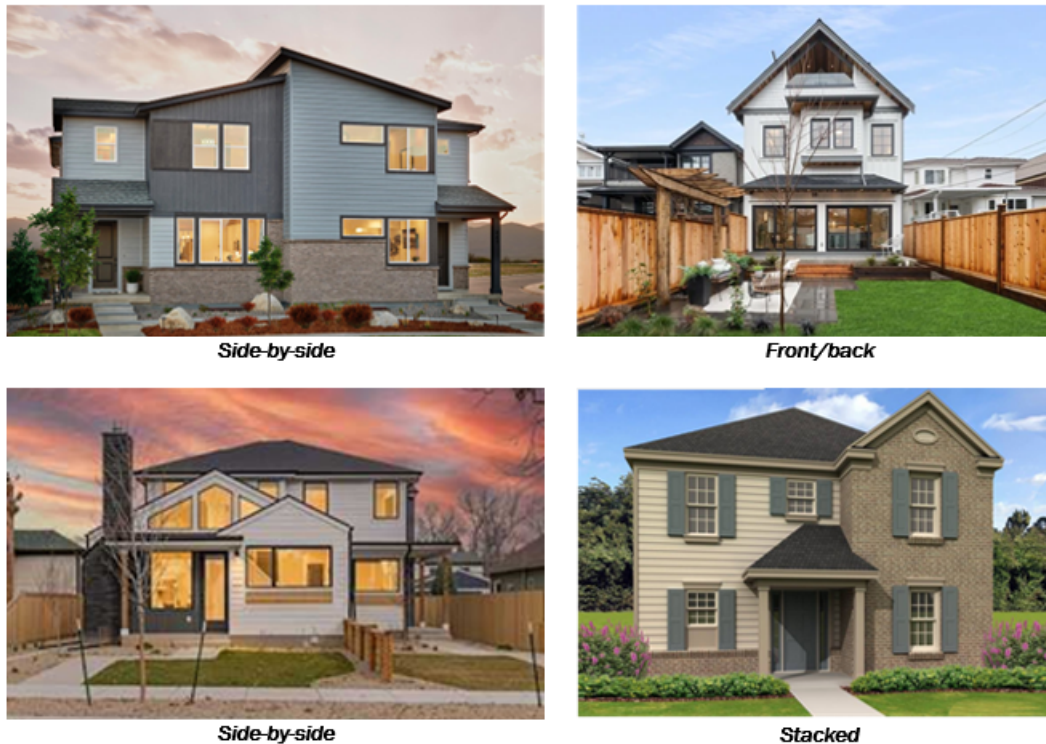
Figure 1: Examples of duplex building forms.
