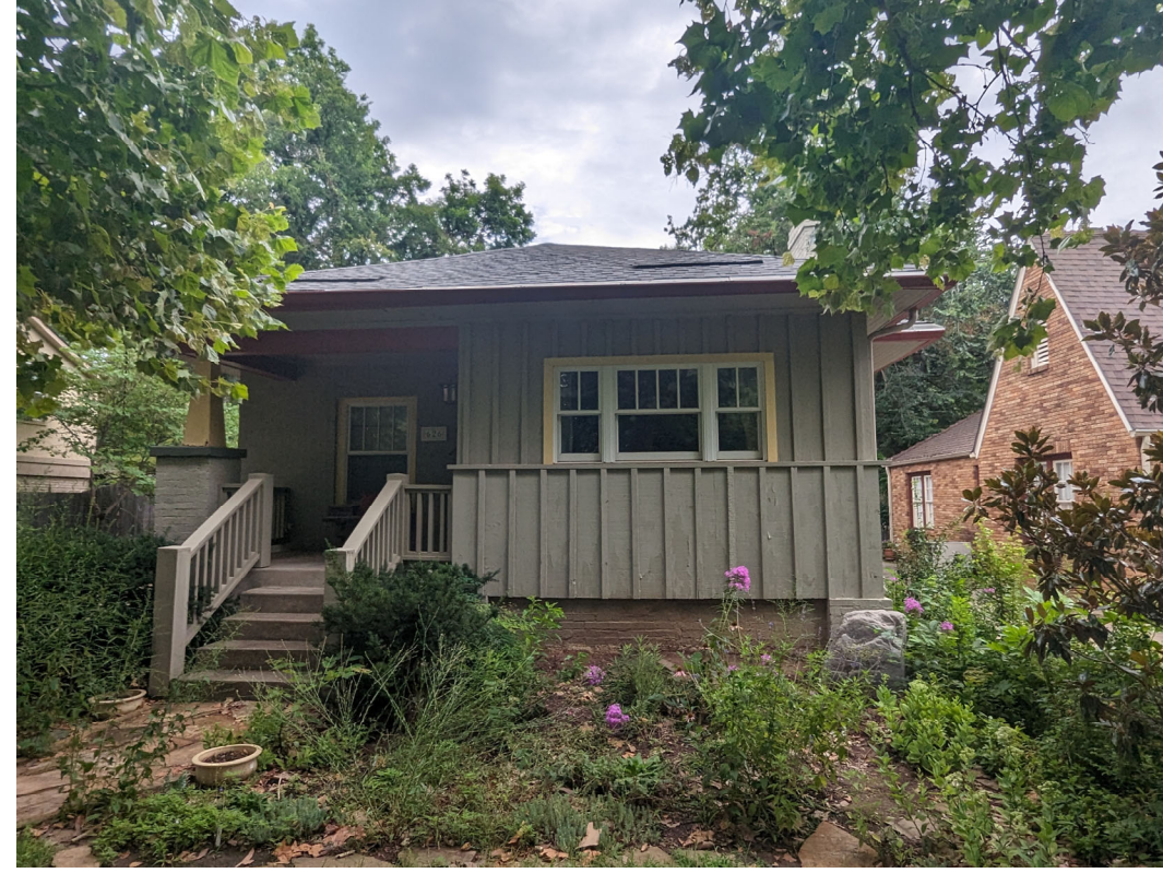
FRONT OF HOUSE (NORTH SIDE)
