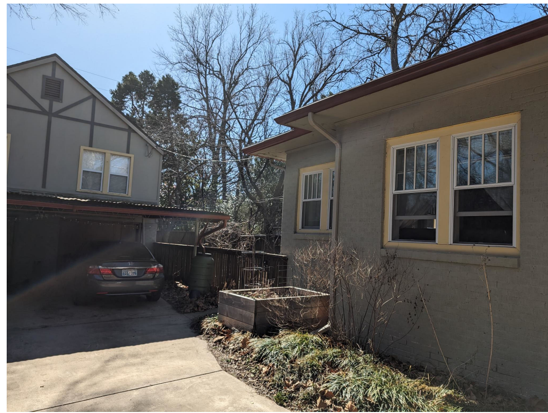
EAST SIDE OF HOUSE/GARAGE (LOOKING SOUTH)
