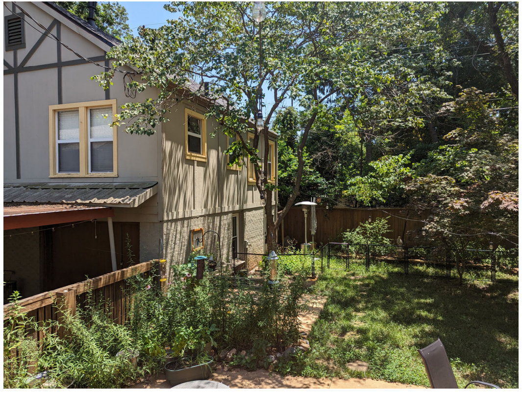
VIEW OF GARAGE (TOWARDS SOUTHEAST)
