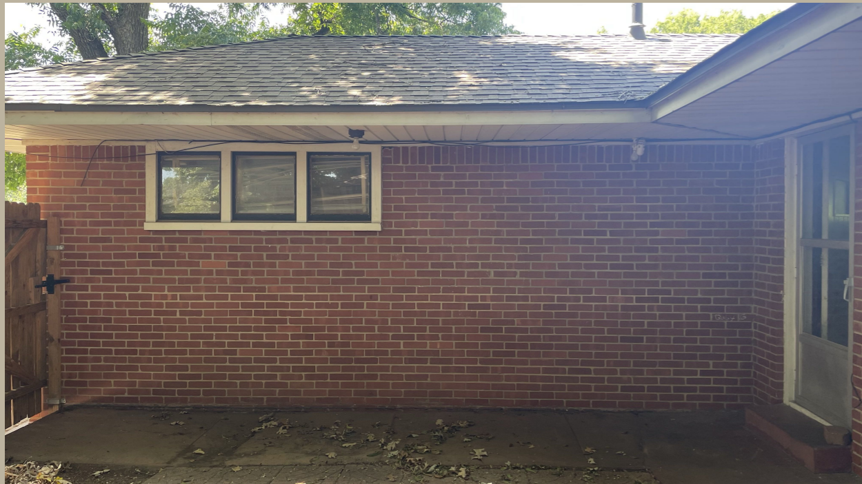
Existing Garage Wall
