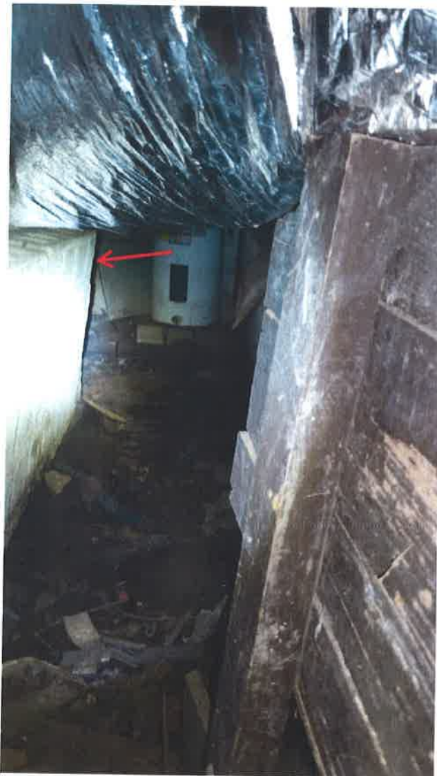
Leaning support wall, moist flooring.
