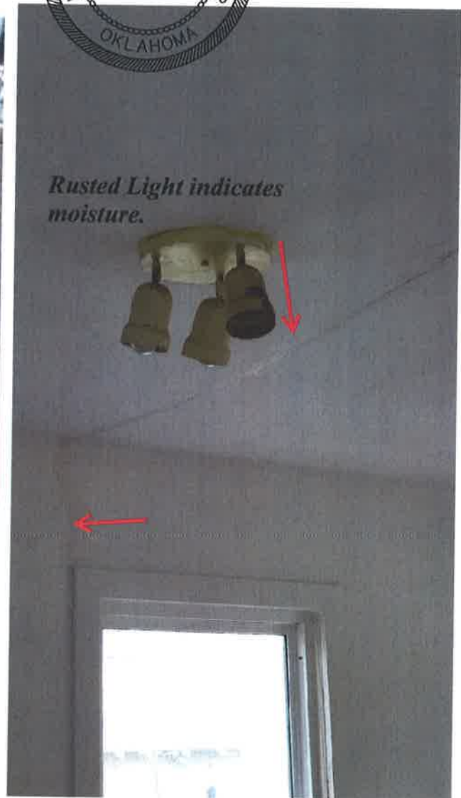
Sagging ceiling and cracks.
