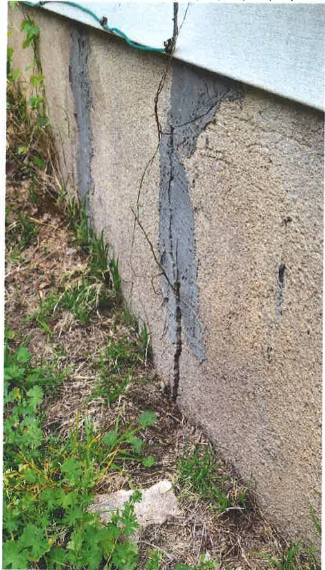
Cracks and displaced stem-wall.
