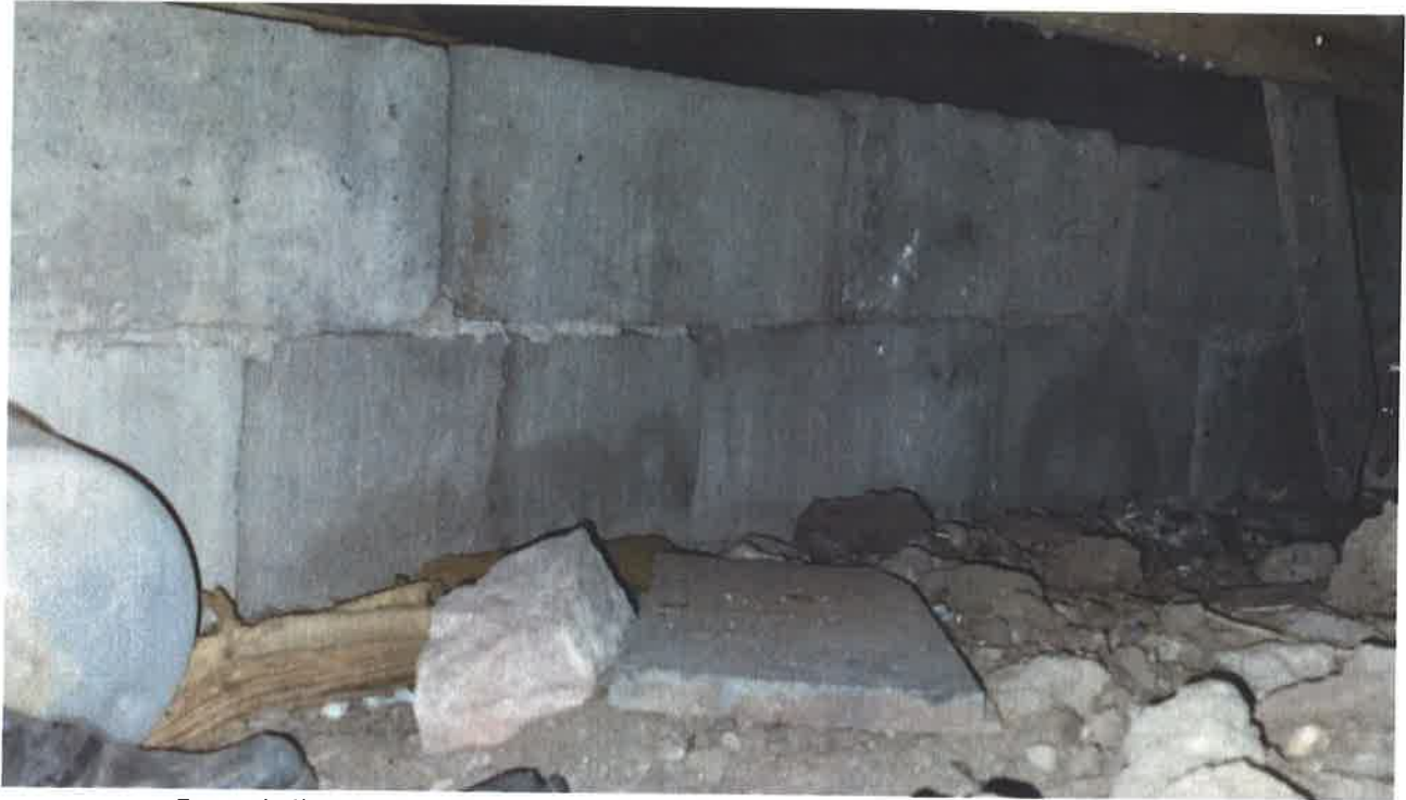
Foundation beneath West End satisfactory (behind basement access).
