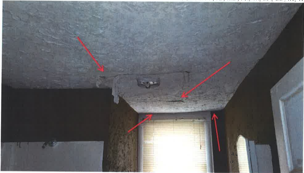
Sagging and crooked ceiling in downstairs bathroom.
