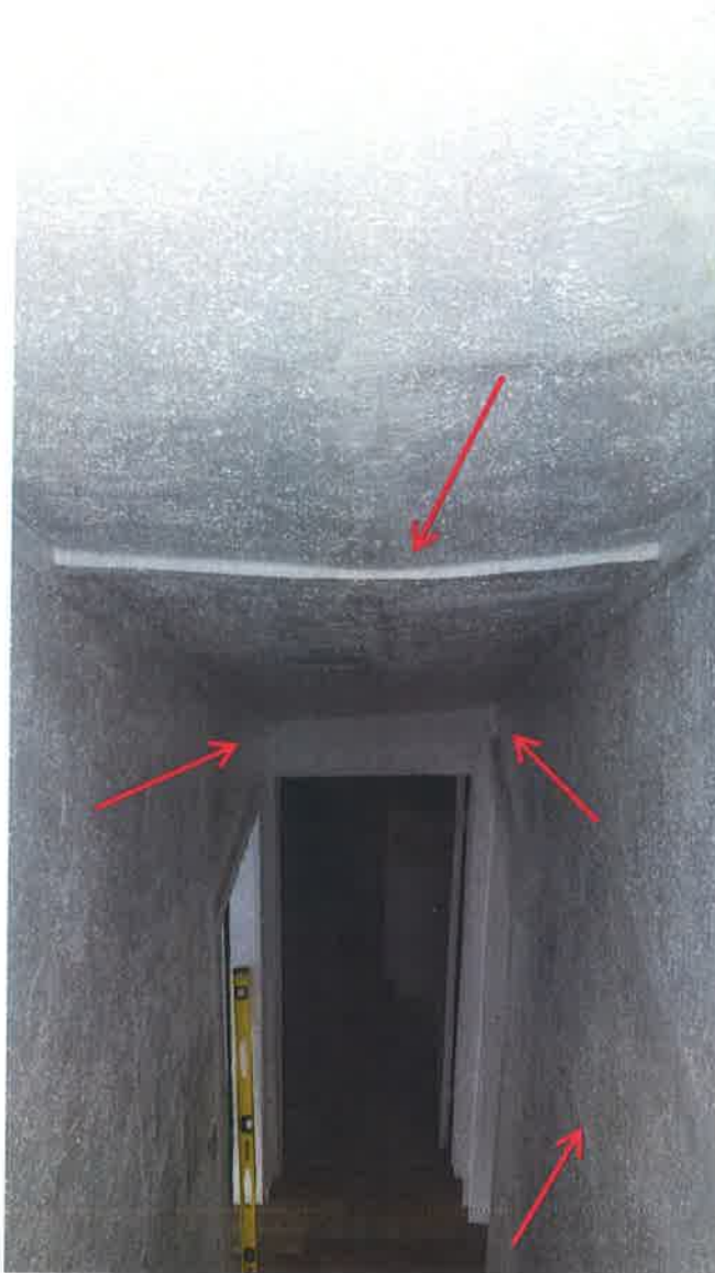
Sagging ceiling in staircase.
