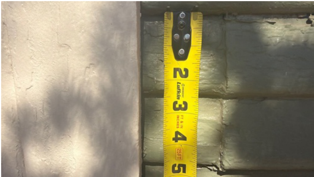
Siding details of existing home
