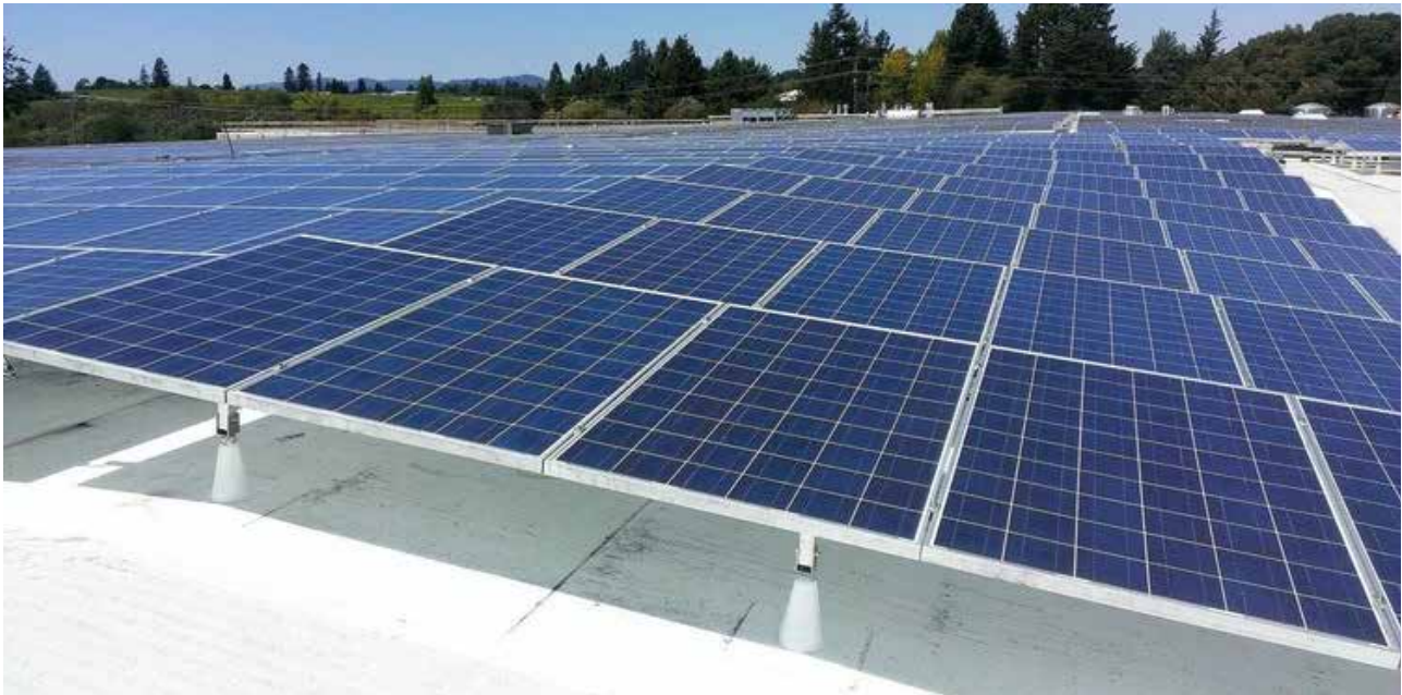
SOLAR PANELS ON LIGHT-COLOR ROOF
