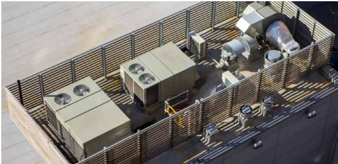
PACKAGED ROOF TOP UNITS
