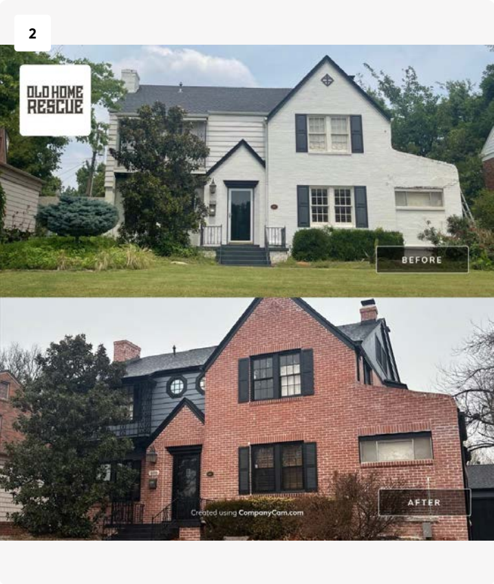
Previous Paint Removal Project • OKC-HP approved paint removal project • Date: 2024 • Location: Crown Heights • Peel Away 7, power washing with low pressure and a 15 degree tip, and the Restorer tool were utilized for the removal of paint
