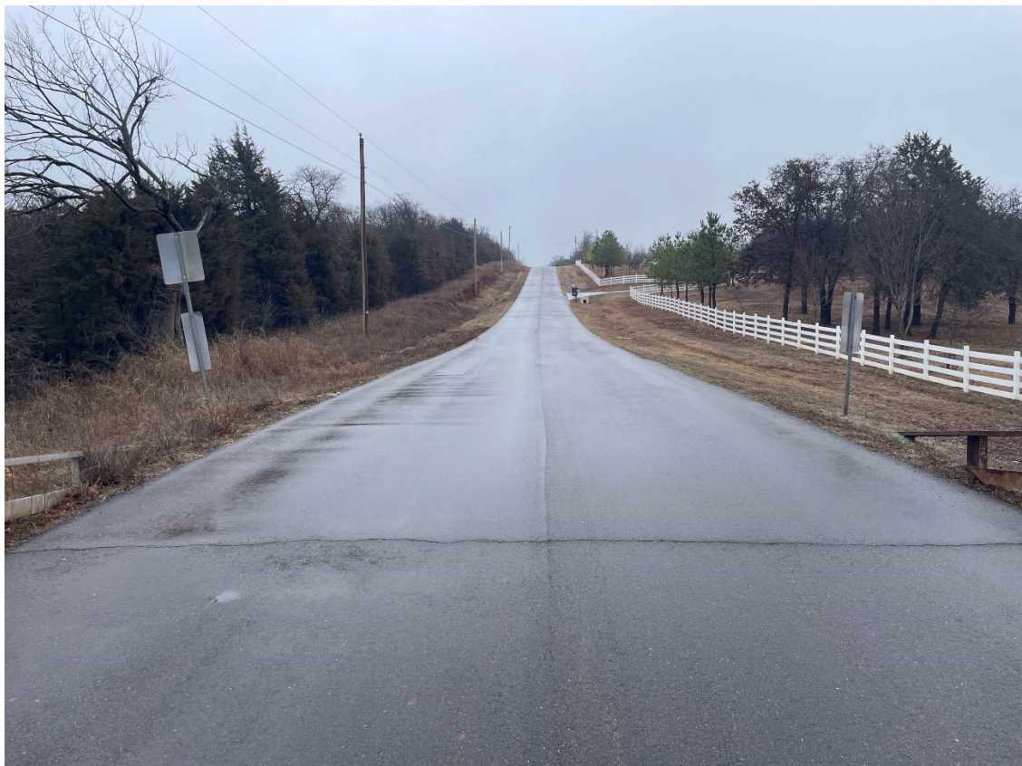
Photo 2. Looking East from Existing Bridge
