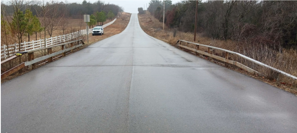
Photo 1. Looking West from Existing Bridge
