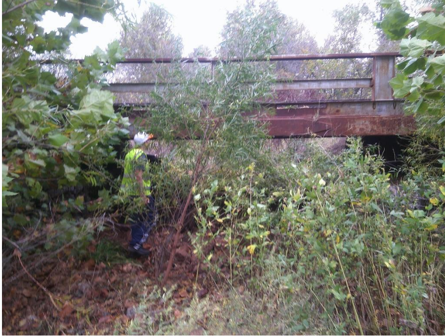
Elevation view, looking north
