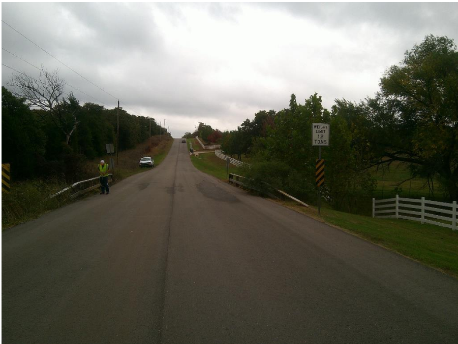
Roadway view, looking east
