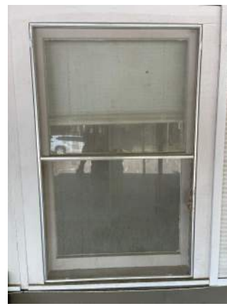
#3. Metal & wood. Does not work. Wood rot.
