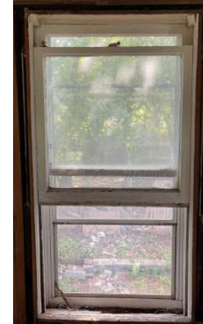
#18. Wood window. Partially working. Wood rot.
