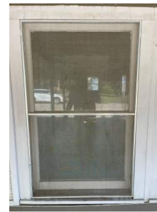
#4. Metal & wood. Does not work. Wood rot.
