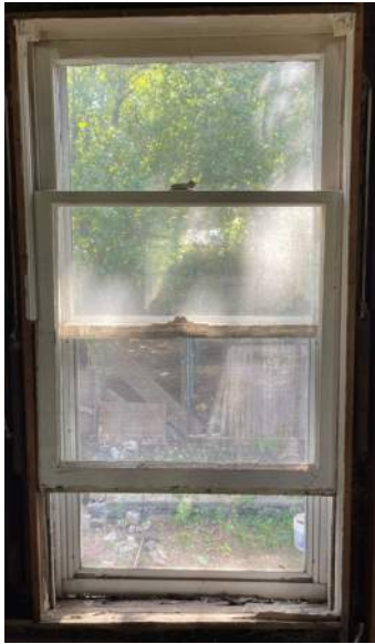
#14. Wood window. Not working, wood rot.
