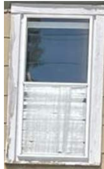
#8. Storm windows over wood-rotten, not working.
