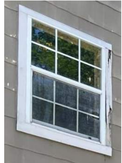
#11. Vinyl window partially working. Wood rot.
