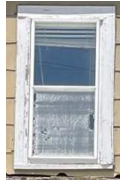
#7. Storm windows over wood-rotten, partially working.
