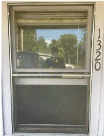
#1. Metal & wood. Partially works. Wood rot.
