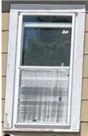
#9. Storm windows over wood-rotten, not working.
