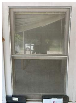
#2. Metal & wood. Partially works. Wood rot.
