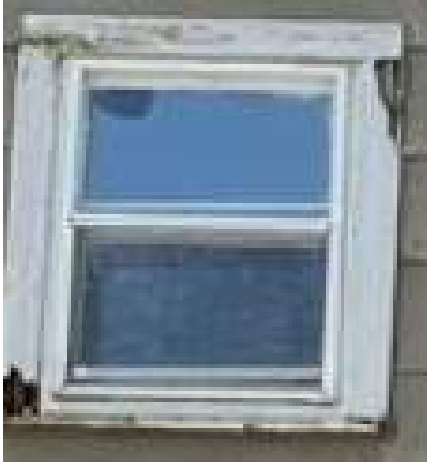
#10. Wood window. Not working. Wood rot.
