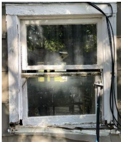
#15. Wood window. Not working, wood rot.
