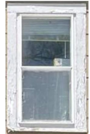
#6. Metal storm windows over wood-rotten, not working.
