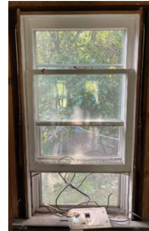
#17. Wood window. Not working, wood rot.
