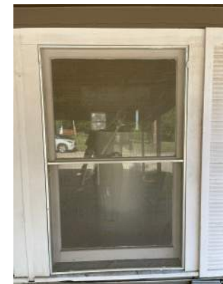
#5. Metal & wood. Does not work. Wood rot.
