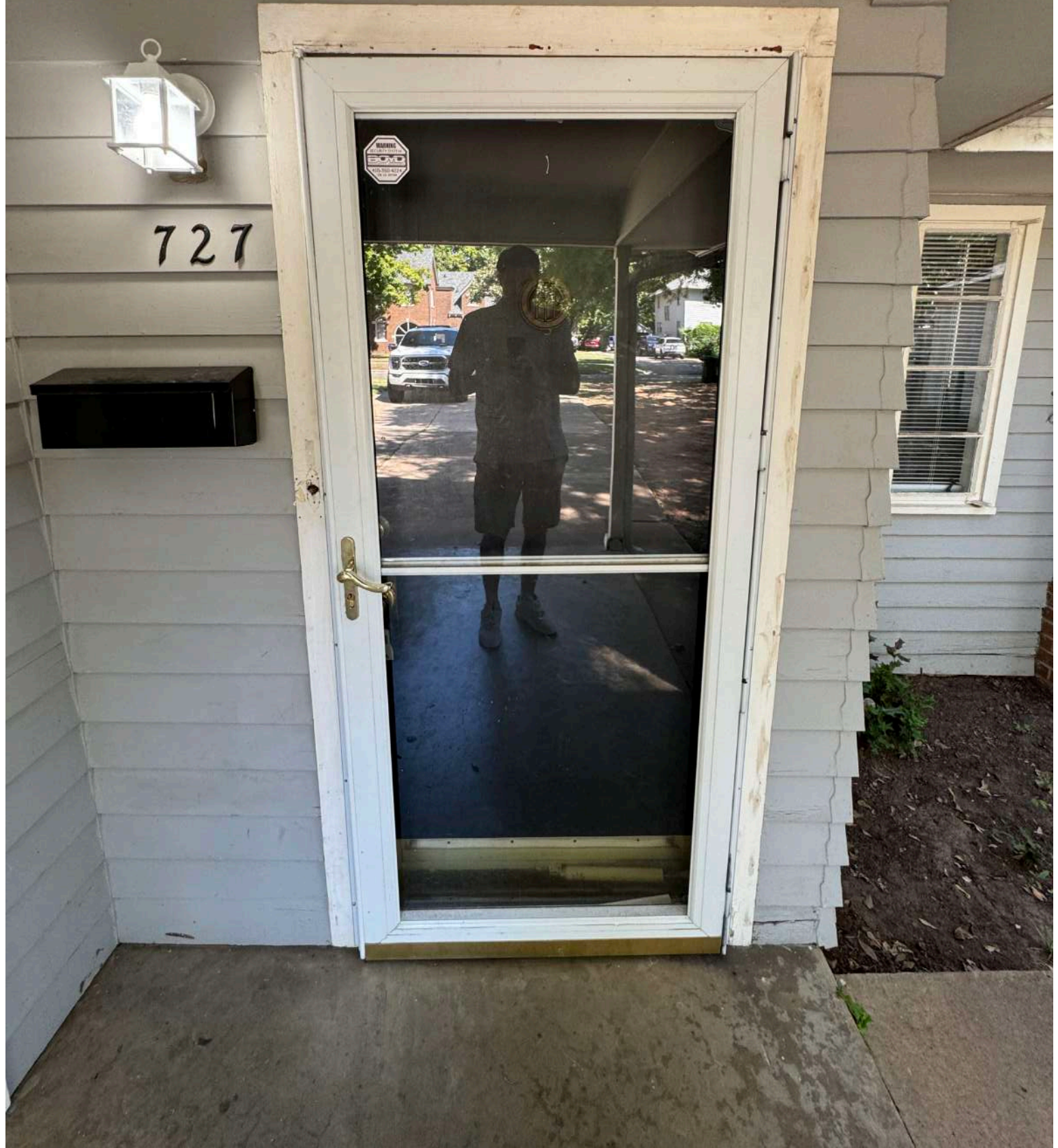
Storm Door at Front Entry
