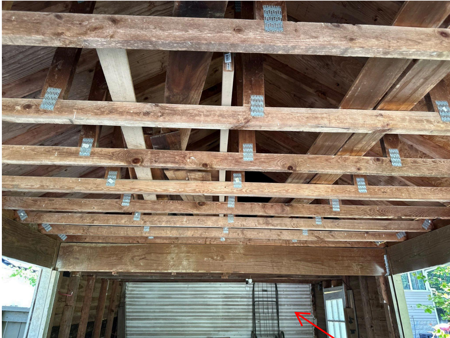
CARPORT "INTERIOR" ROOF STRUCTURE
