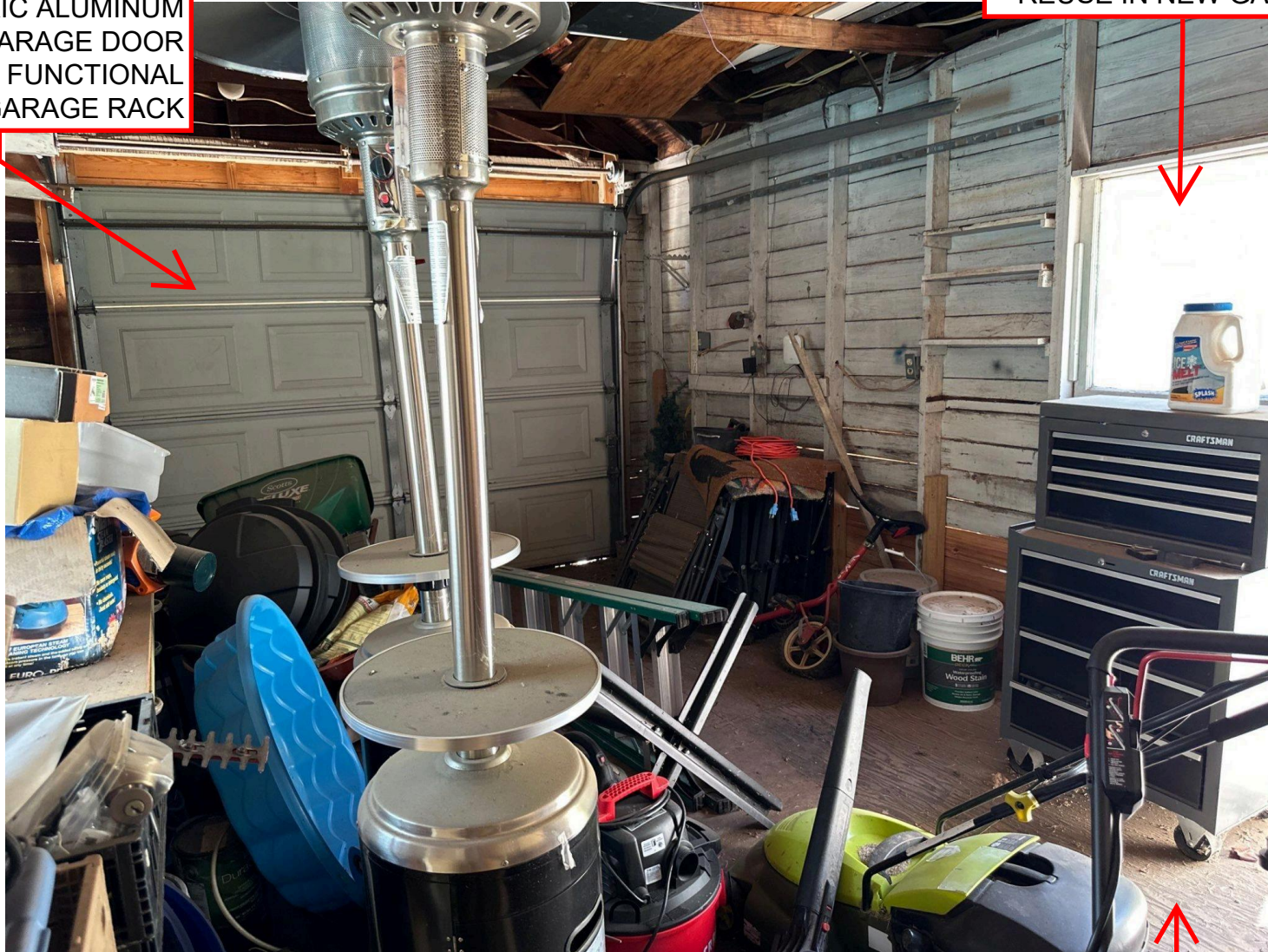
GARAGE INTERIOR LOOKING EAST-SOUTHEAST
