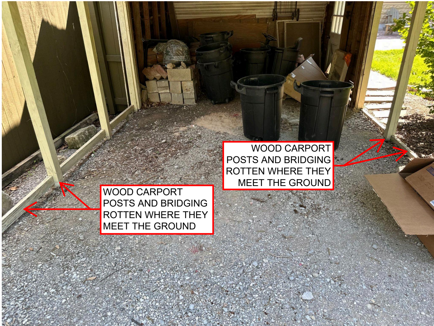
CARPORT "INTERIOR" GRAVEL FLOOR
