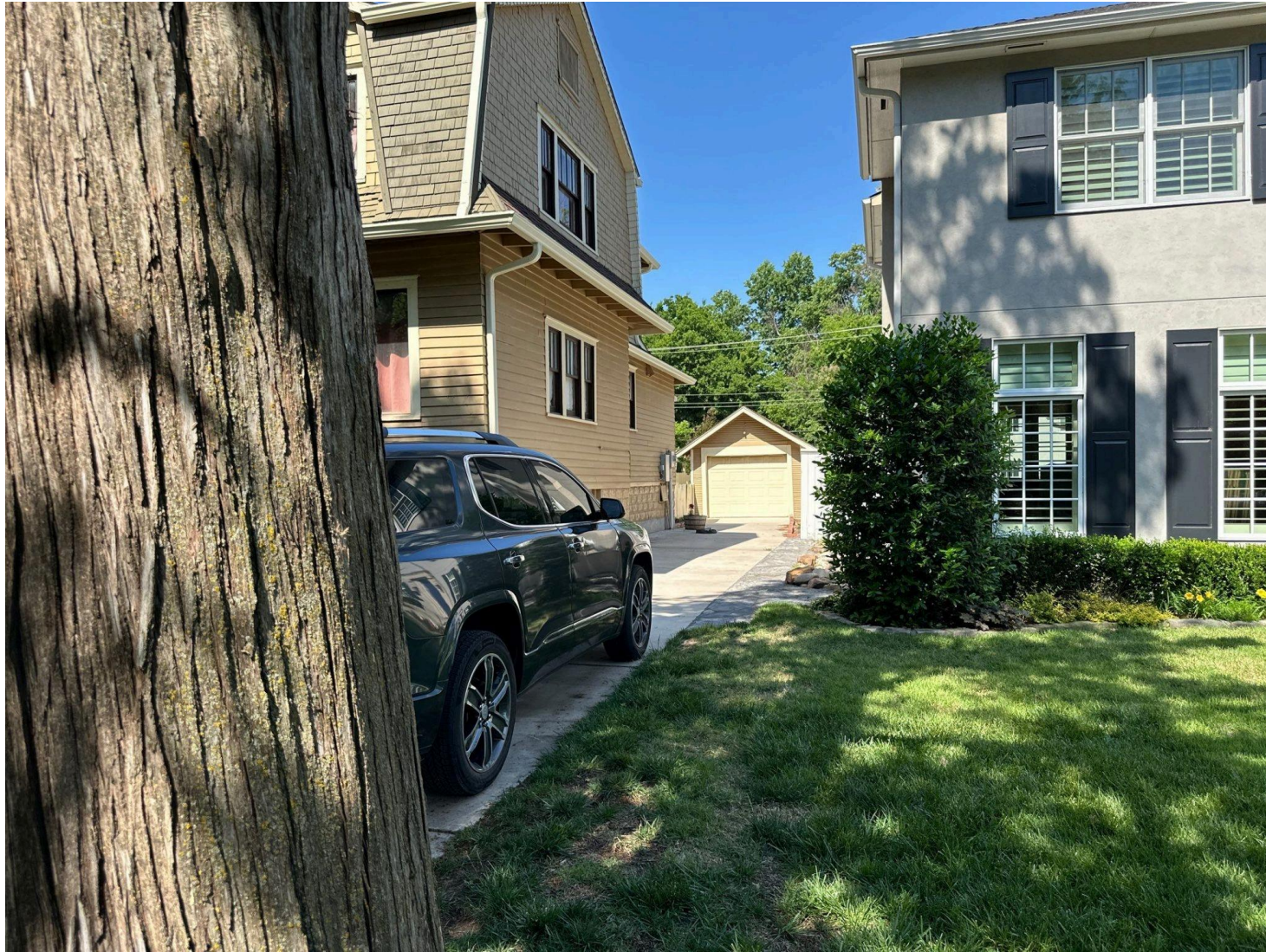
VIEW OF EAST (FRONT) ELEVATION OF GARAGE FROM PUBLIC RIGHT-OF-WAY
