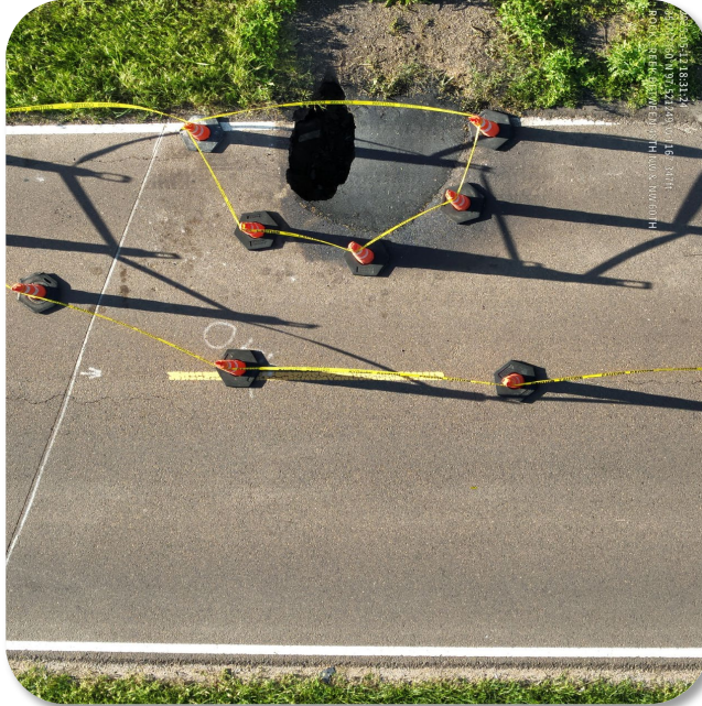
Large Void on Rock Creek Road and 60 th Avenue NW
