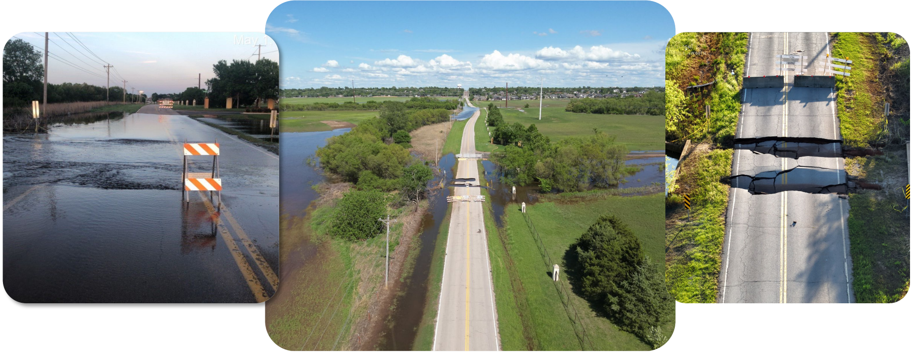
Road Failure Robinson Street between 48 th Avenue NW and 60 th Avenue NW
