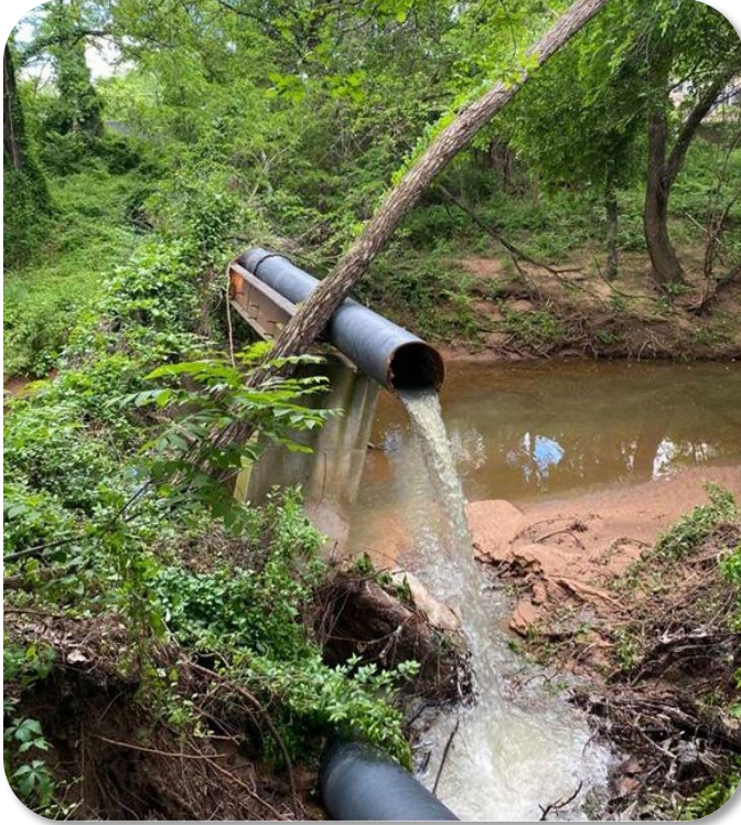
Sewer Failure near 730 Stinson Avenue
