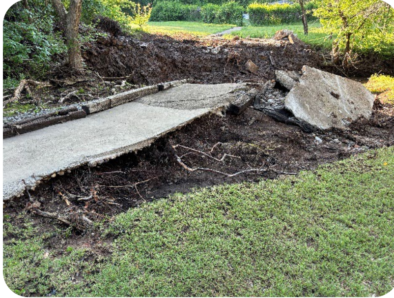
Brookhaven Creek Pedestrian Bridge Collapse
