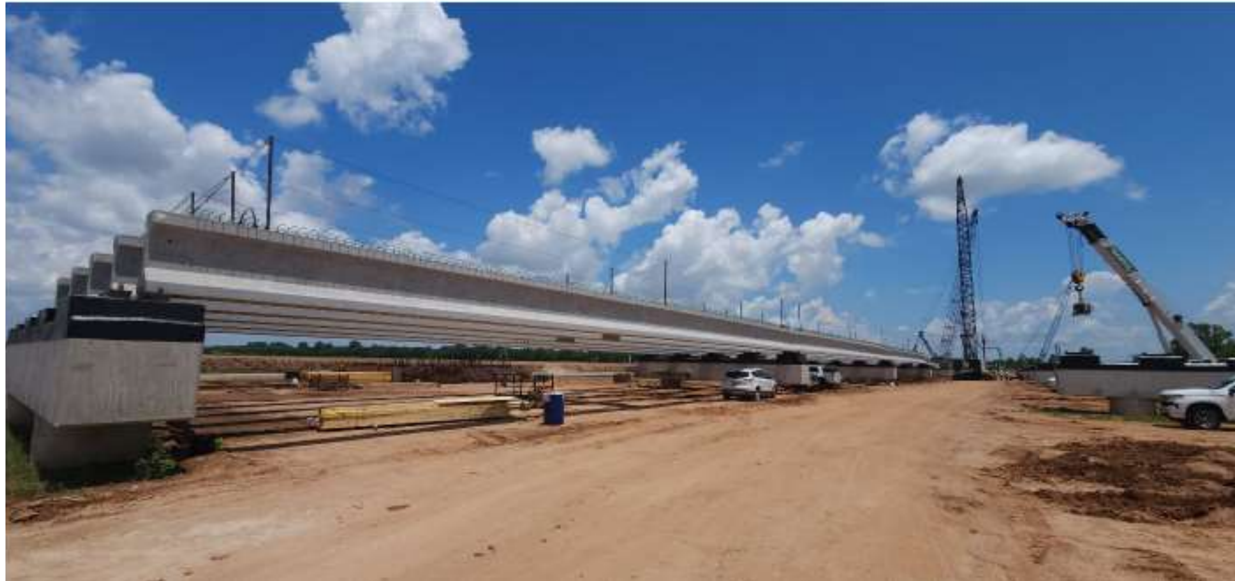
Eastbound and westbound bridges over 10-Mile Flats Creek 0.15 miles east of Pennsylvania Ave. extending east Bridge beams set into place.
