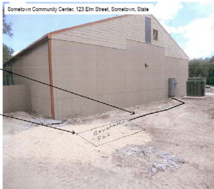
Figure 4. Ground-level photograph showing proposed ground disturbance area.
