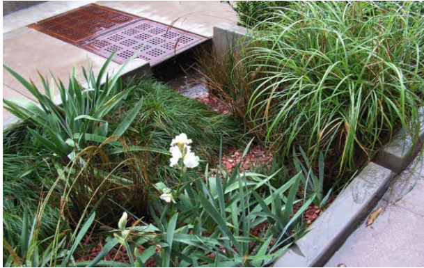
Swale with curb cut opening and decorative grate outlet (Credit: AHBE Landscape Architects)
