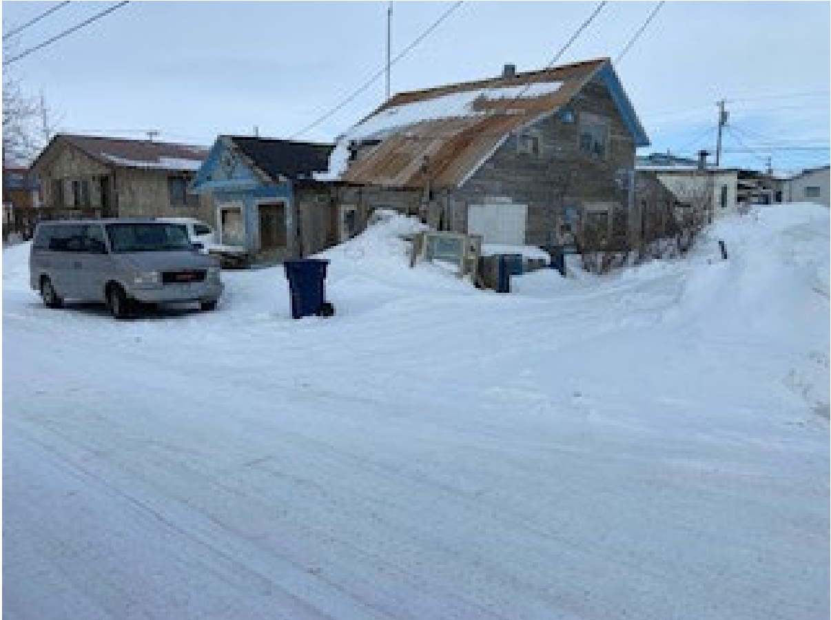
108 East King Place – Randall Spencer – 001.161.15
