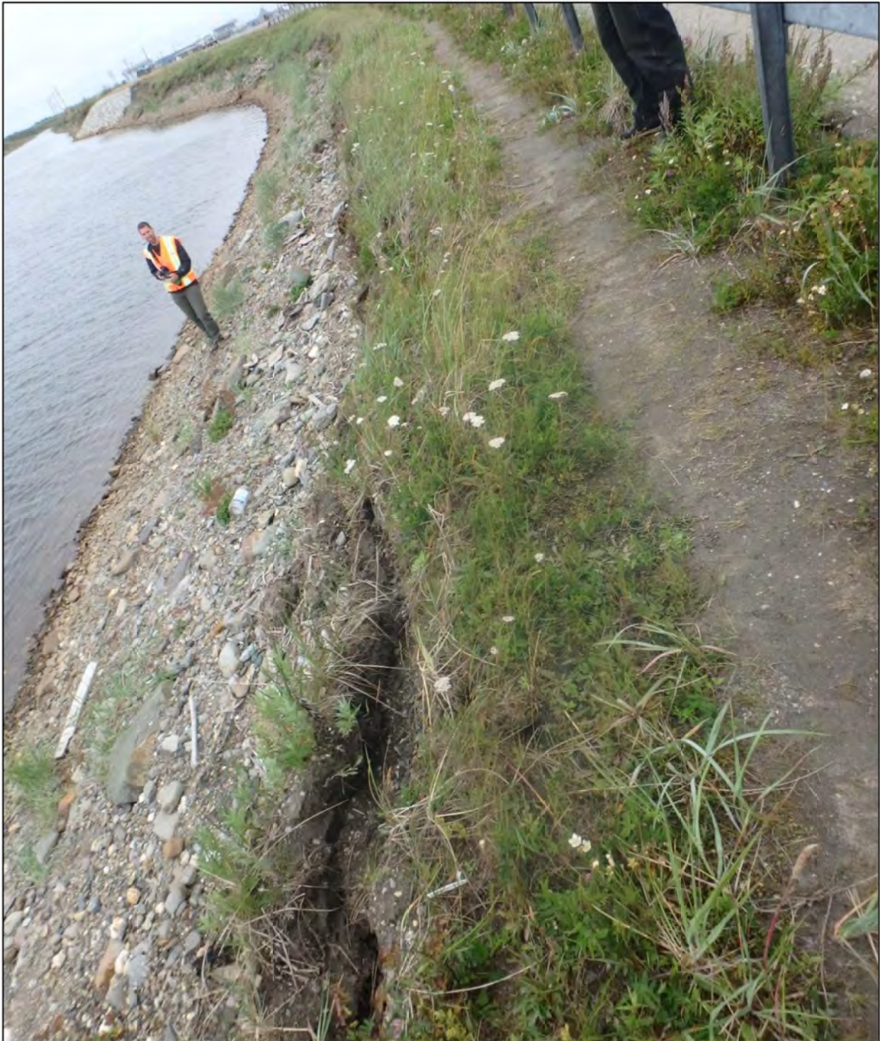
Figure 2. Tension crack at top of Snake River bank, upstream of new bridge. PDC Engineers photo.
