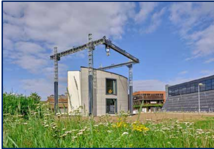
Figure 17: Example of Gantry-Style Printer
