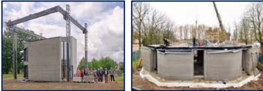
Figure 1: Construction 3D Concrete Printing
