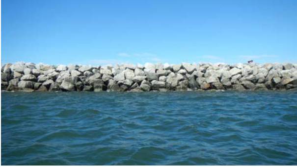
Causeway revetment
