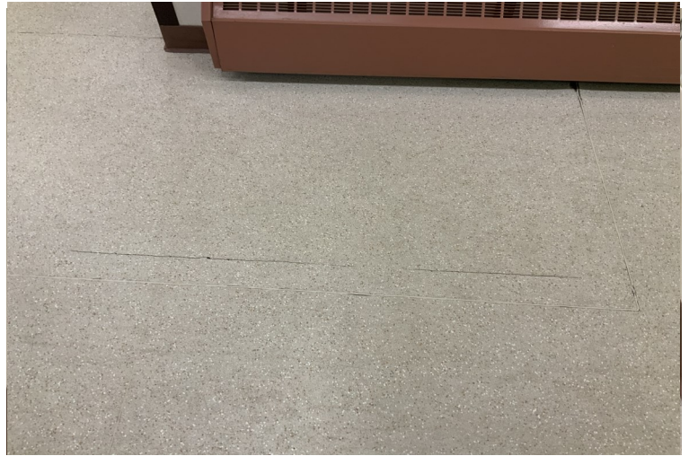
Old Worn Flooring: Heavy traffic and repeated use have led to cracks forming on the floor of the women's locker room. As the degradation continues water will seep down into the subfloor.
