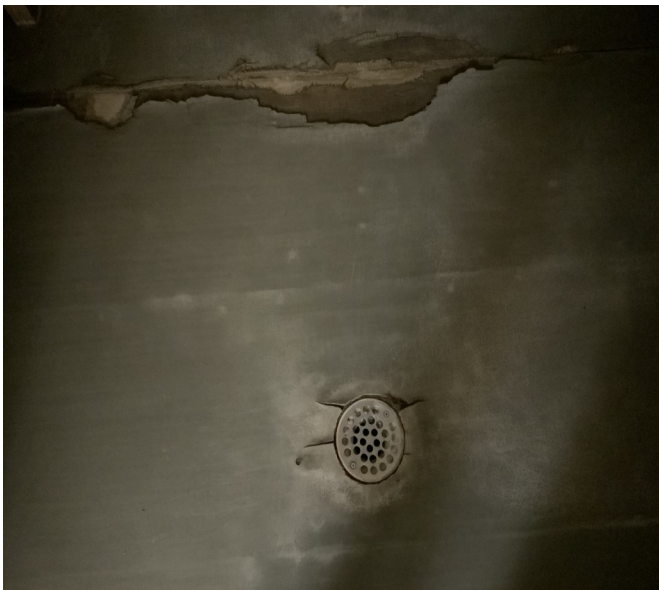
Compromised Floor in Men's Sauna: The last time the men's sauna floor was fixed it was not graded to drain properly leading to failure in the flooring seams. Once water began to get underneath it the floor began to peel.
