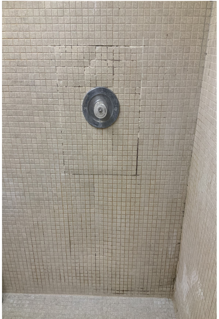
Needs Immediate Attention: Water has permeated the tile in the women's group shower so thoroughly that the walls are collapsing as evidenced by the wavy pattern visible above. In the lower right corner it is completely rotted.
