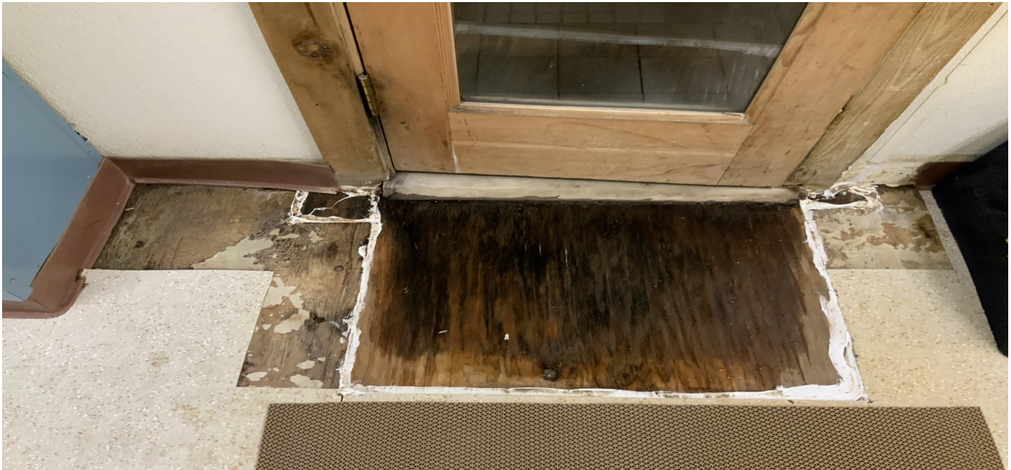
Beyond Repair: Years of water flowing out of the women's sauna has rotted the threshold, flooring and sub-flooring. As patrons need to step on this area to enter the sauna there are major safety concerns regarding the possibility that the floor will collapse causing potential injury to a patron.
