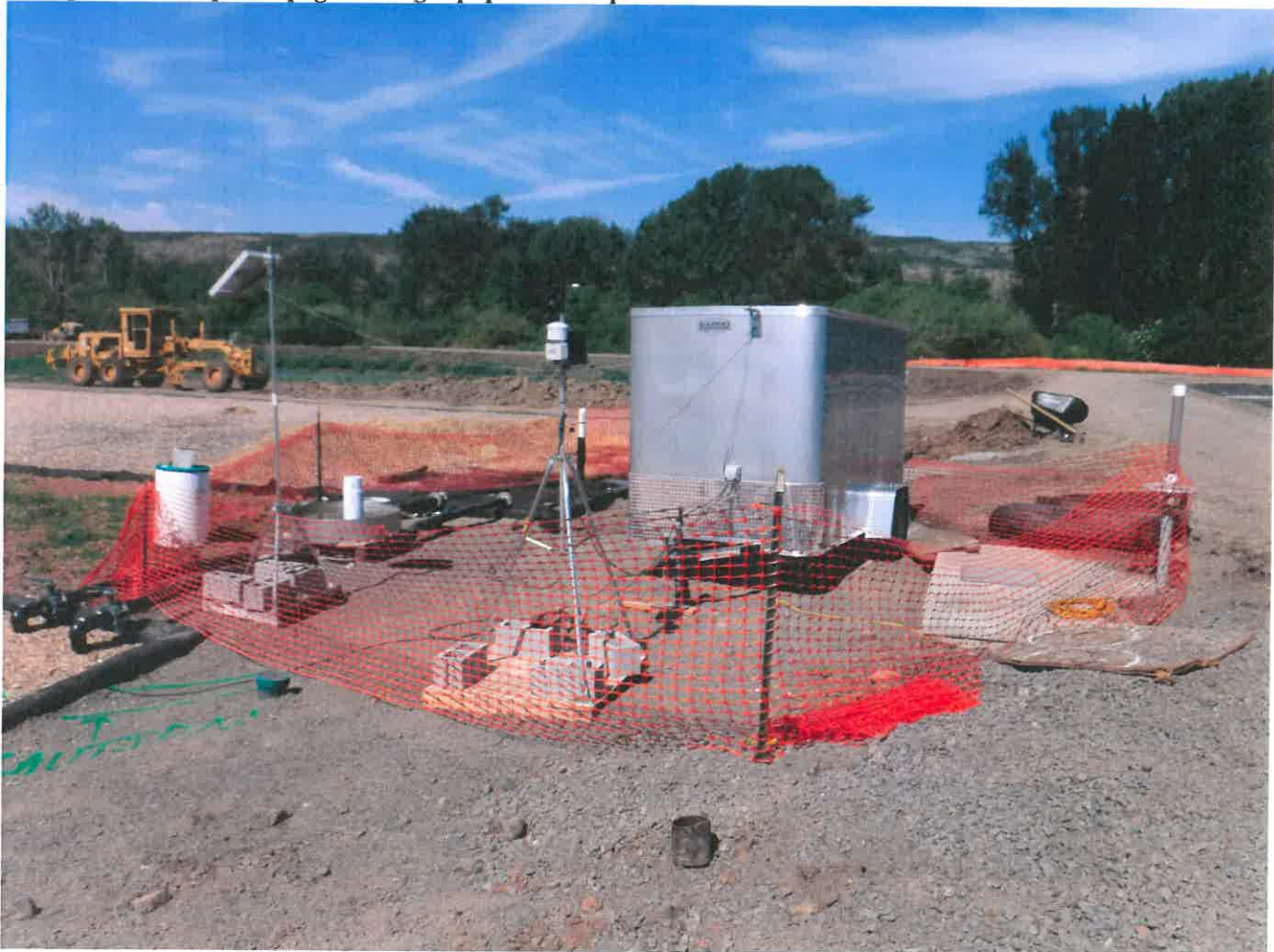
Figure 1: Example Seepage Testing Equipment Setup
