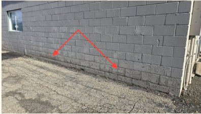
failing paint
