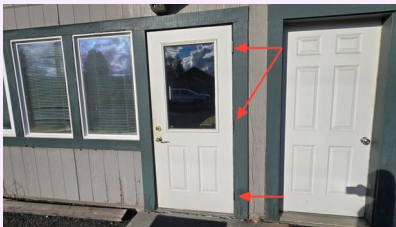
removeable hinge pins
