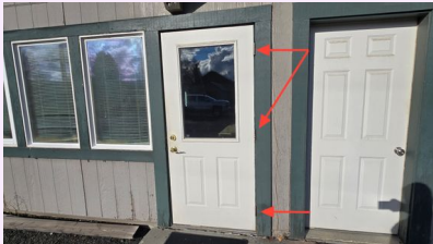
removeable hinge pins
