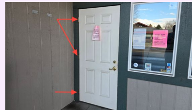
removeable hinge pins
