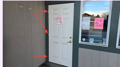
removeable hinge pins
