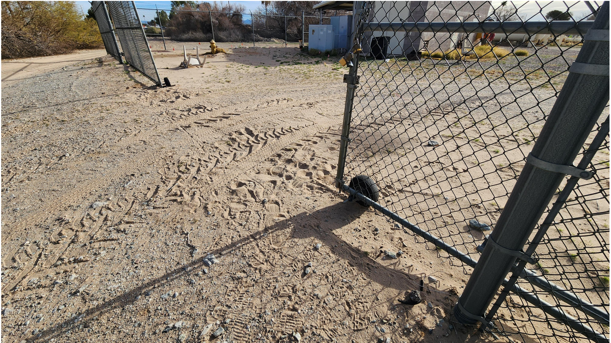
Existing 30-ft wide entrance gate with rubber wheel rollers (exterior rollers missing)
