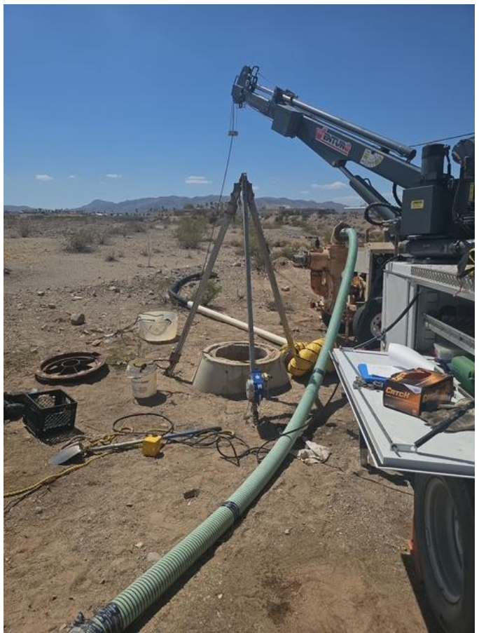
Hospital Gravity line cleaning, temporary bypass pumping, and debris removed
