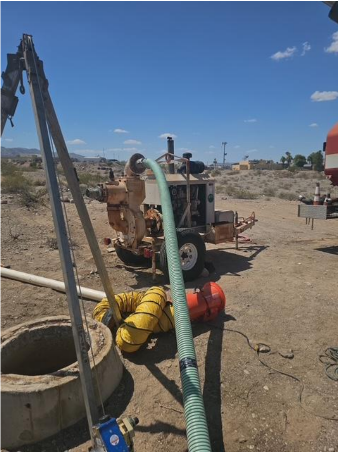
Hospital Gravity line cleaning, temporary bypass pumping, and debris removed
