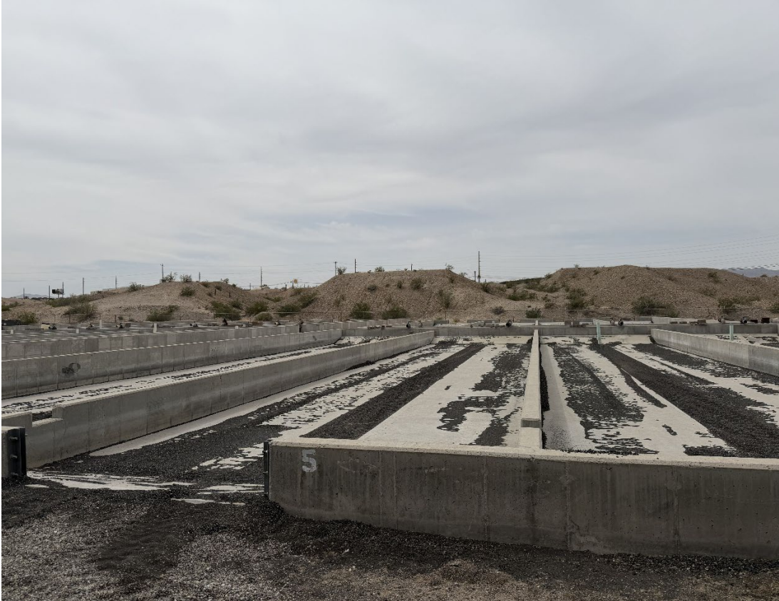
Figure 16. Sludge drying beds. There are a total of twenty-four sludge drying beds onsite.
