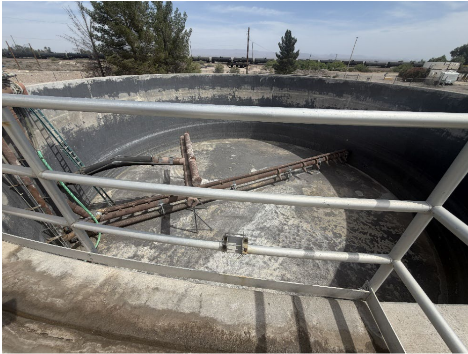
Figure 7. SBR No. 2 not in operation due to yearly maintenance. Typically, one SBR is in operation at a time.
