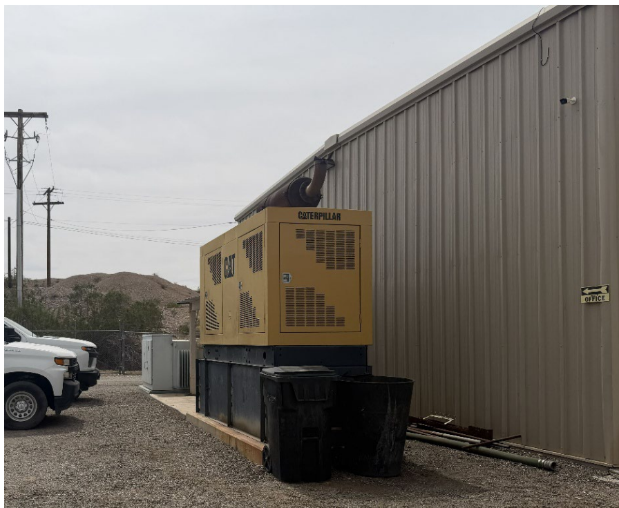
Figure 10. The emergency generator provides power to run the Facility in the event of a power outage.
