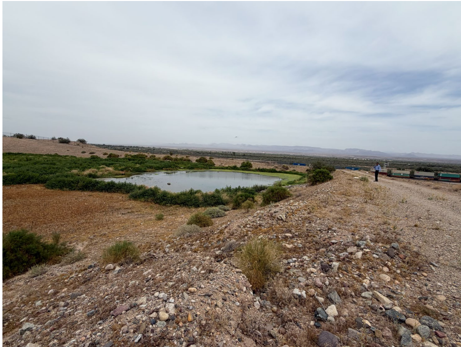
Figure 19. Evaporation/percolation Pond No. 2 was the only pond receiving treated wastewater flows at the time of inspection. Approximately less than a quarter of the pond was observed to be filled with treated wastewater.
