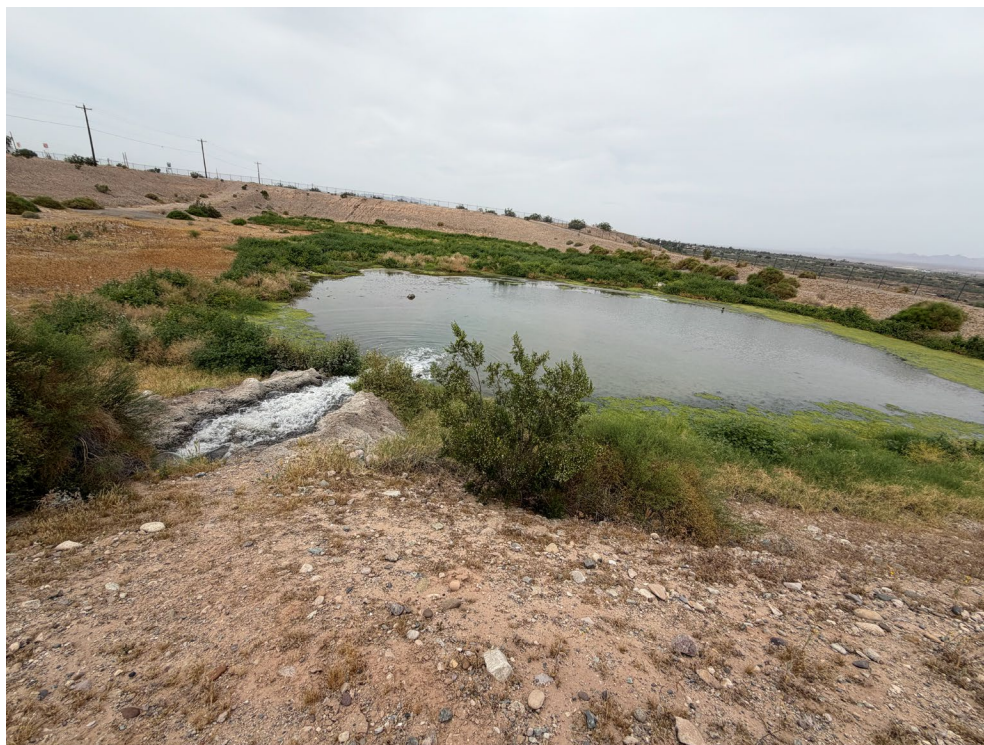
Figure 20. The influent pipe to Evaporation/percolation Pond No. 2 was observed.
