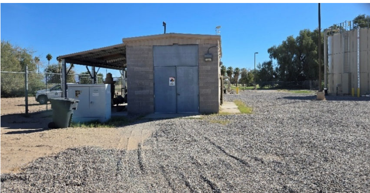
New Treatment Facility
