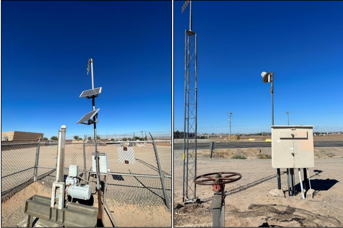
Electronic gate control and metering stations.
