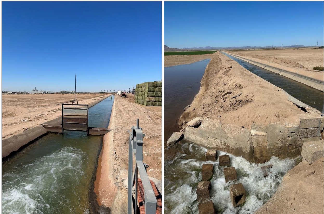
Water flowing down a concrete-lined ditch (left), water running out of a high-flow concrete farm turnout (right).
