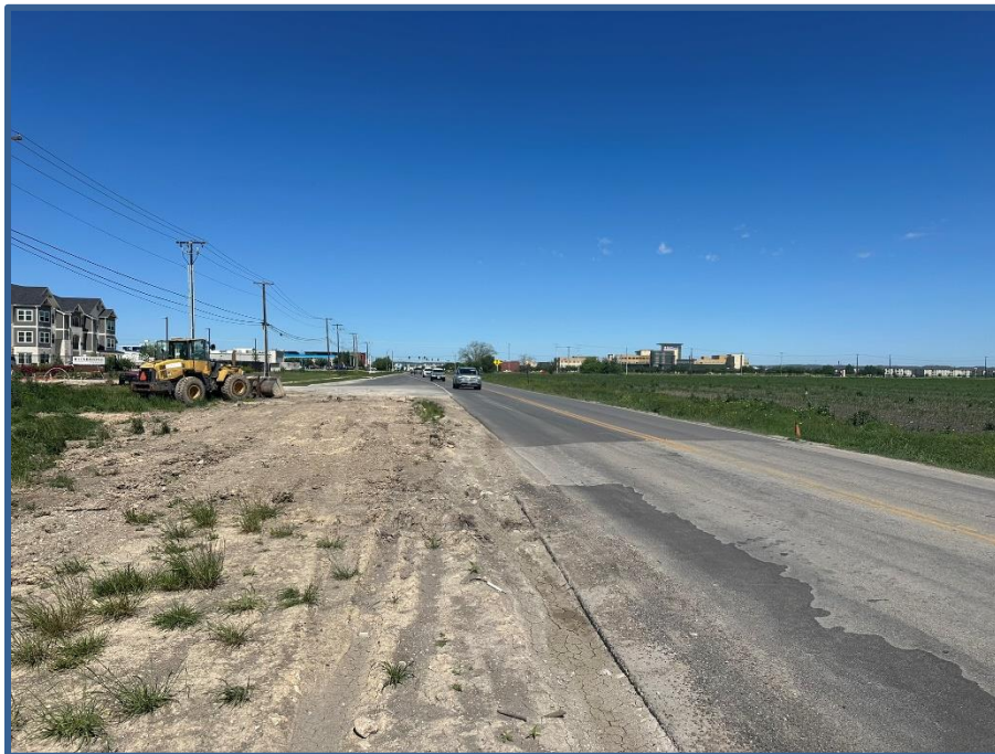
View looking northwest along Barbarosa Road. The subject property is on the left.
