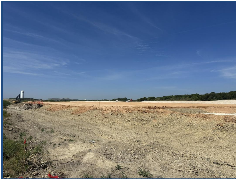
View looking at proposed substation site on the middle portion of the subject property.
