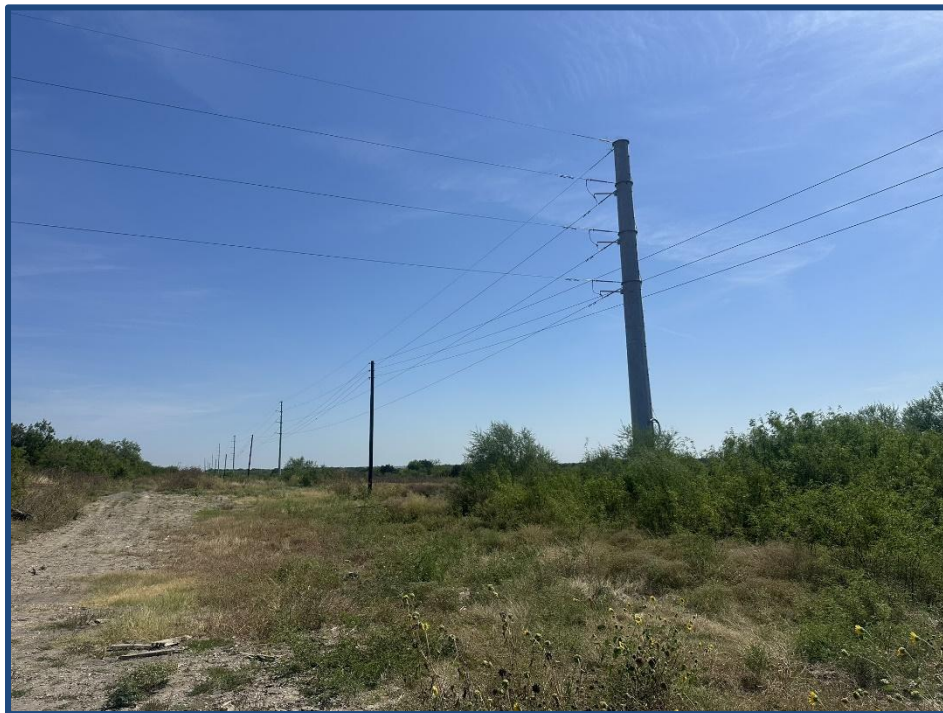
View of existing transmission line along the eastern property boundary.
