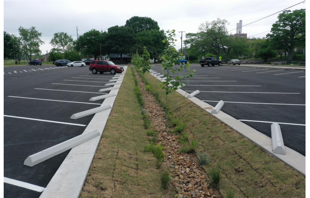
Biofiltration System located at Landa Park Aquatic Center
