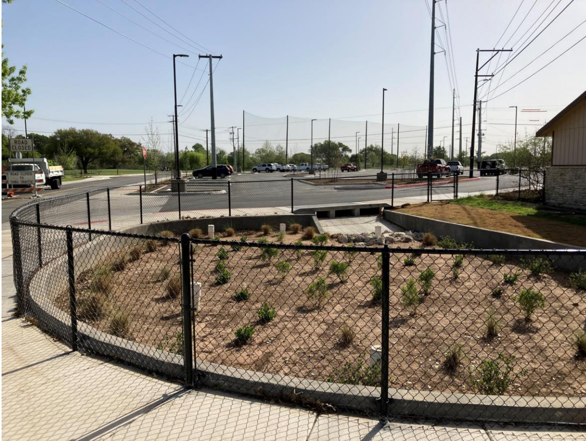
Biofiltration system located at Elizabeth Ave. and Landa Park Dr.
