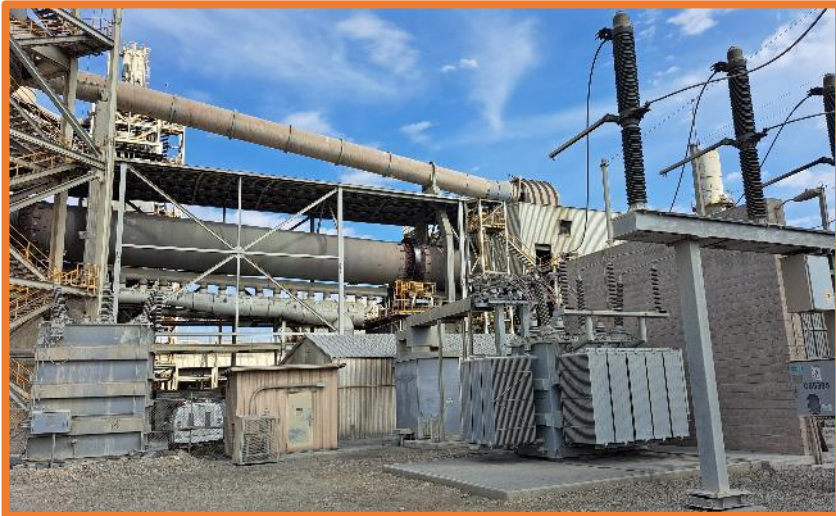
Industrial Substation PWT Replacement, TXI T1 ($1.1M)
