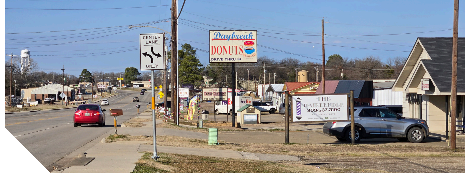
Northbound view of Highway 37
