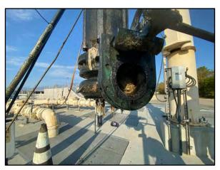
Staff installed the new replacement grinder for the belt press. The grinder helps protect the Seepex sludge pump and cuts up rags so they do not get stuck within the belt press.
