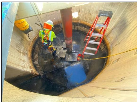
Staff had All Valley Crane come out to pull out the auger at the headworks to replace the brush on the auger. While the crane was here, staff replaced the spider couplings in aerators 8 through 11 on aeration tanks 4 and 5.
