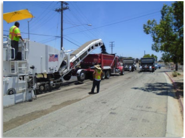
City of Calimesa | Citywide Pavement Rehabilitation
