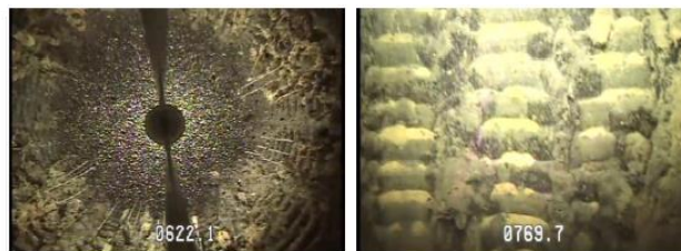
Figure 5 – Encrusting and biological material on well screen.
