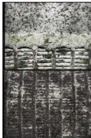
Screened intervals 690 ft and 800 ft BEFORE chemical treatment.
