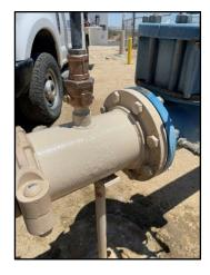
• Well 31 Pump Noise – The pump was removed from this well and was inspected for necessary repairs. Additionally, since the pump was out of the well, we conducted a video survey and EMDS (well casing study) on the well. It was determined that all the downhole equipment needs to be replaced. The new equipment installation was completed on June 25, 2024. Staff are working on collecting the necessary water samples to put this well back online.
