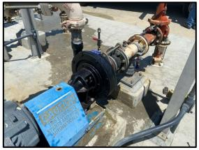
One of the speed reducers that drive Clarifier 3 failed and needed to be replaced. Staff is working with Nord to locate a new gearbox as a replacement. Until then, staff has isolated flow away from Aeration Tank 3 and sending it to Aeration Tanks 1, 2, 4, and 5. Aeration Tanks 4 and 5 are taking most of the flow.
