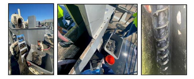
Staff replaced the upper and lower doctor blades for the belt press. These blades clean off the sludge of the belts into the auger for disposal.
