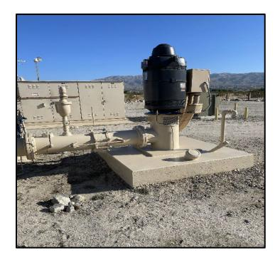
• Well 29 Production Meter – Staff replaced the production meter on September 26, 2023. The meter that was removed will be sent to McCrometer for recalibration.
