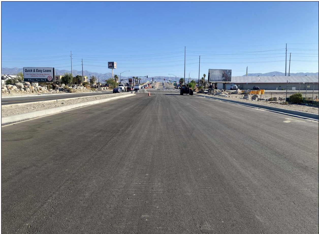
Figure 34. Segment of Indian Canyon Drive in the APE (Site 33-008410), south of Garnet Avenue. (Photographs taken on June 18, 2025; view to the north)
