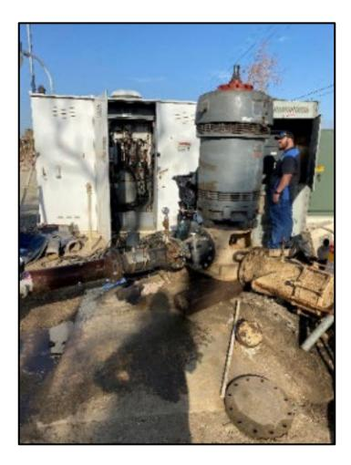
Staff replaced the shaft packing on the Two Bunch Booster 1 due to excessing leaking.
