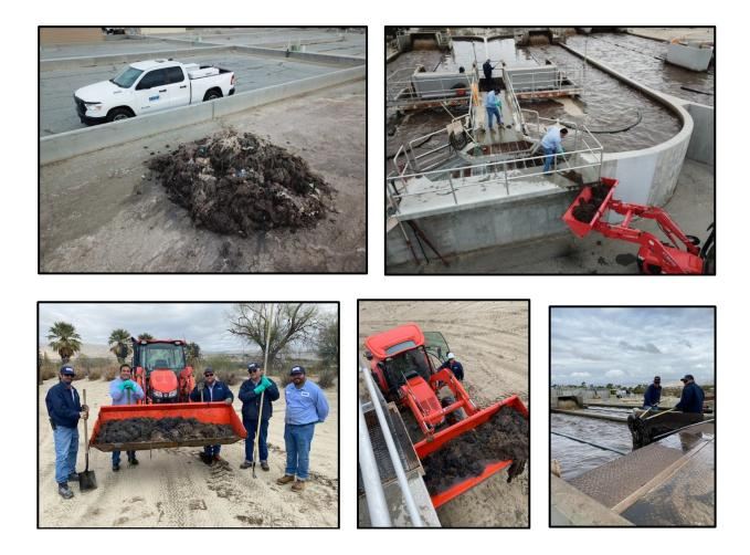
Clarifier 2 was having issues with constant rising denitrified sludge. Staff drained the tank to clean out any septic sludge and grit on the bottom of the clarifier. Upon inspection of the tank, one of the support rods for the lower sweeps had broken off due to corrosion. Staff was able to make a temporary fix until this tank can be taken offline and fully rehabilitated. The rod was held up with 304 stainless steel chain, nut, and bolts to keep it approximately 1/2 - 3/4 inches off the ground.
