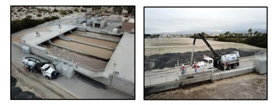
Due to increasing solids and regular rainfall throughout the past months, staff helped with vacuuming wet sludge out of the wasting beds as the Desert Crest WWTP. The rain and cold weather has prevented the sludge in these wasting beds from drying.
