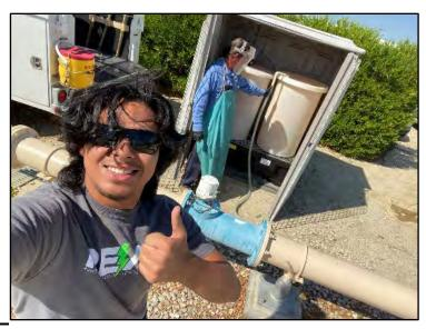
Well 26A – Staff replaced the packing in the downstream OS&Y valve on the backflow prevention assembly for the uranium filtration plant.
